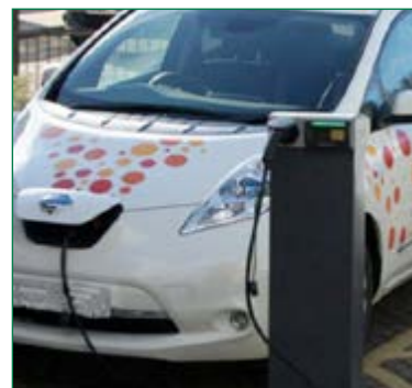
Installing electric vehicle charging
