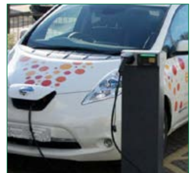
Installing electric vehicle charging
